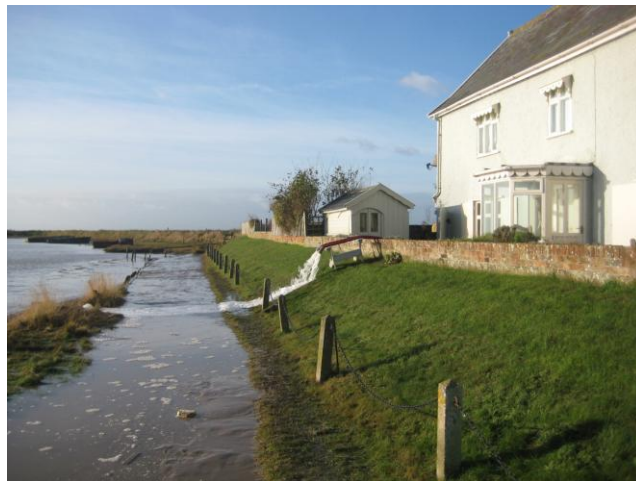
Pumping out Quay House Garden
