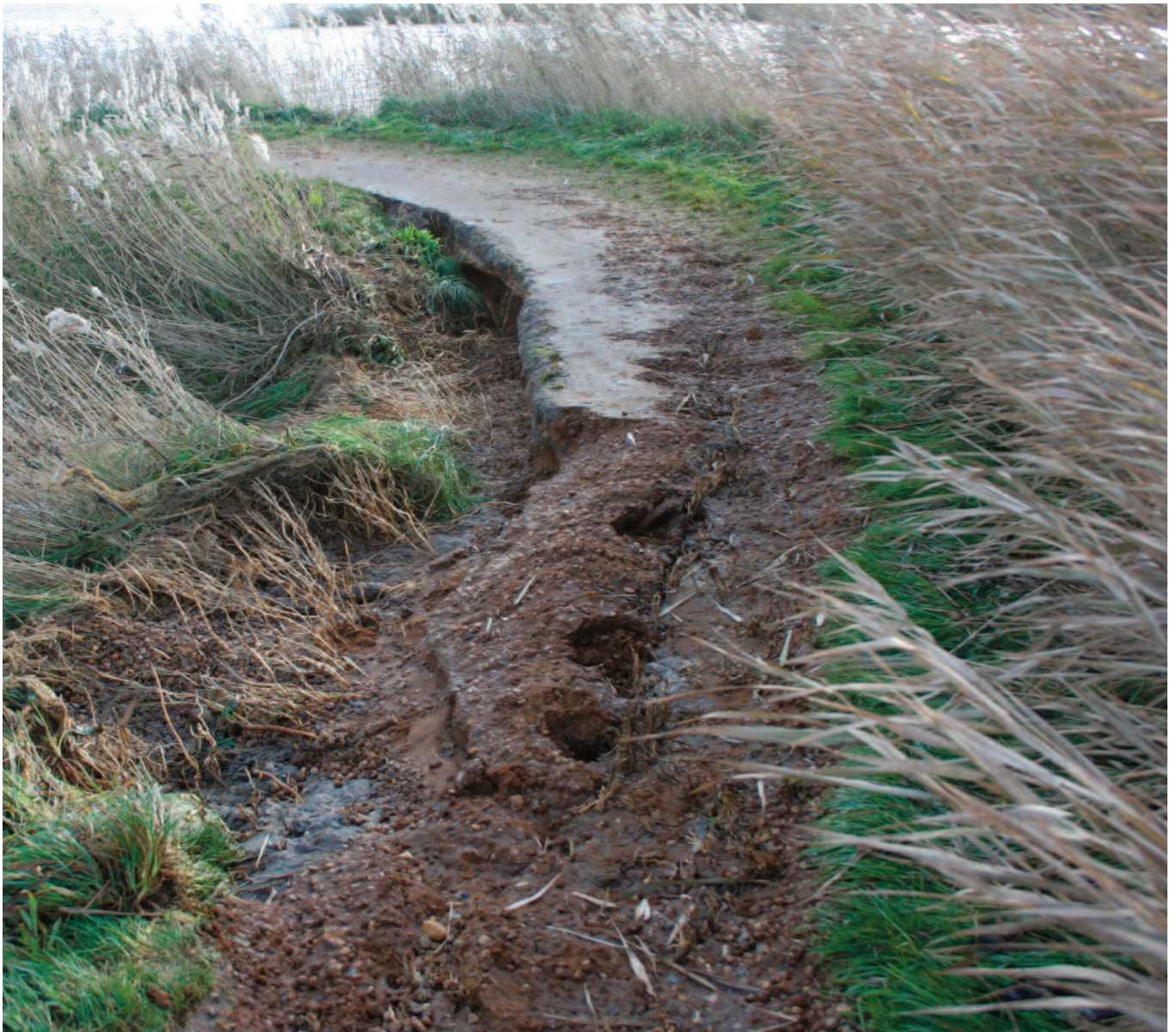
The bend at TM 3969 5752 shows the most serious collapse with the inner grass bank collapsed and the hoggin path starting to be undercut.
