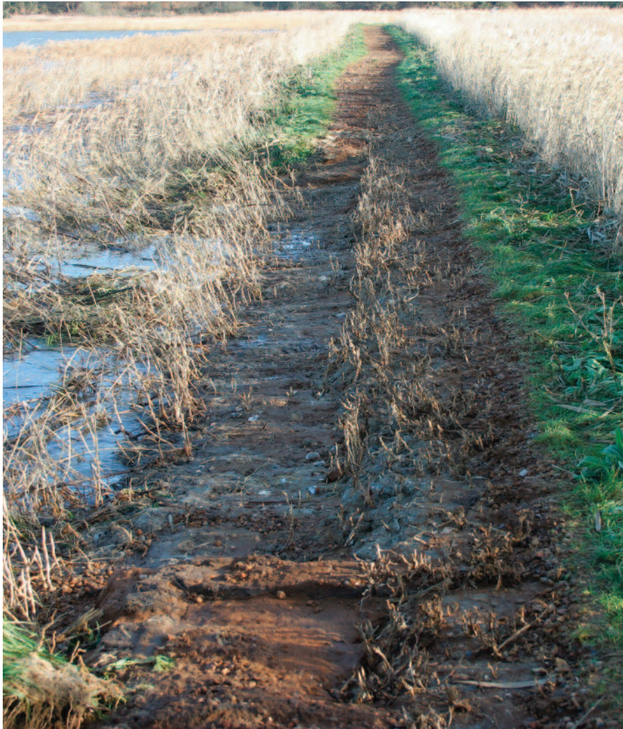
in places the inner grass bank has collapsed with the hoggin sucked away
