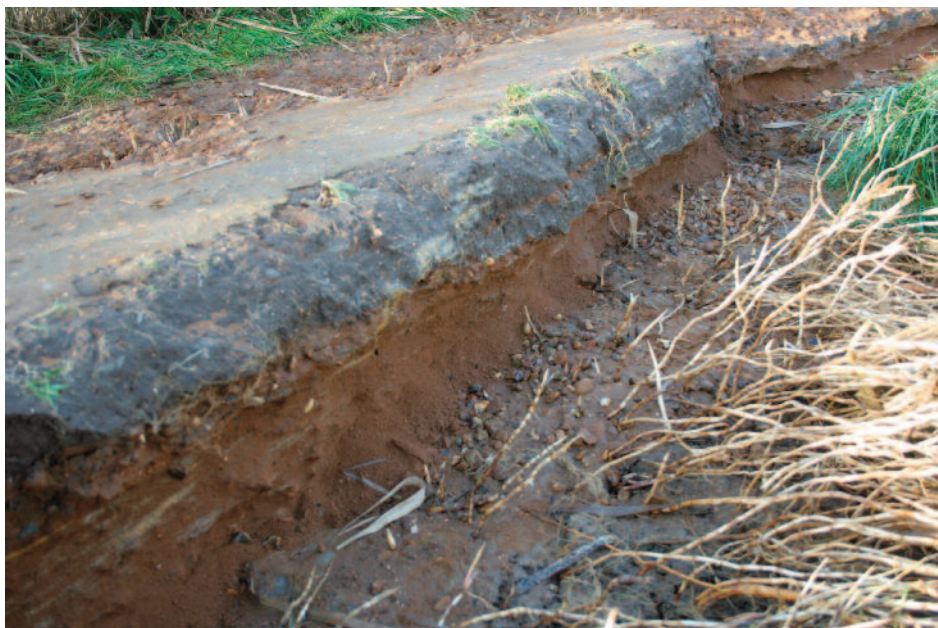
The bend at TM 3969 5752 shows the most serious collapse with the inner grass bank collapsed and the hoggin path starting to be undercut.
