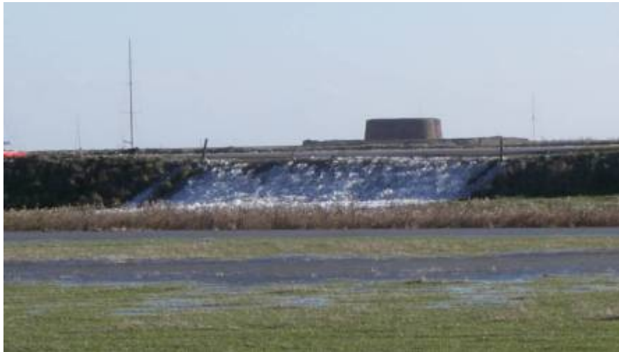
Overtopping on Aldeburgh River Wall – photo courtesy of Andrew Hawes November 2007
