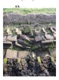
2. Map ref 458557 East of Aldeburgh Sluice, one 10 strides from where 2011 wall re- armoured, the worst patch is a further 4 strides and has clay wall exposed to water at every high tide see photos
