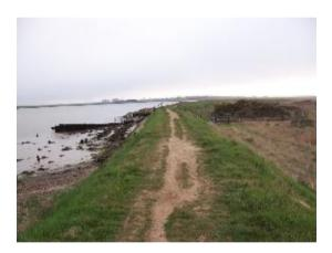
4. 460558-460556 between sewage works and Slaughden road, the path has more than doubled its width from the old boarded track, query is the wall being trodden lower by moving outwards?
