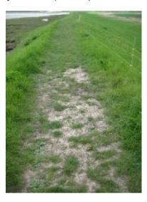
9 18 mtrs of erosion above the revetments 100 mtrs from Cordle Boundary (424491)
