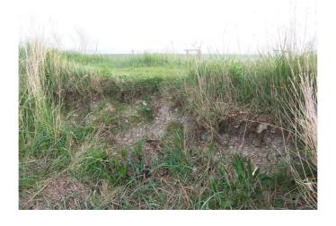
**B2. Rear of bank at Aldeburgh pump.** The land behind continues to remain muddy and wet long after all other parts of the walls have dried out. There is evidence of slumping near the base, hidden in the vegetation. (recently cleared by EA to get a better look which is good)
