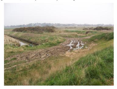
**B.3** Slumped wall on the most walked stretch between Slaughden and the steps TM 460558 This part was overtopped in the December 2-13 surge. It dips below the rest of the wall and suffers a lot of heavy walking wear.
