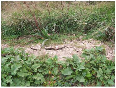
**A.4 near vertical back/land ward slope of almost 1/5th of a mile of river wall TM445561 - 459564.** In some places, in the distance on the photo below, the slope :height of bank ratio is near to 1 in 3 and clearly while there is some grass there are bare patches which would not withstand overtopping, just as steep slopes failed at Hazlewood marshes
