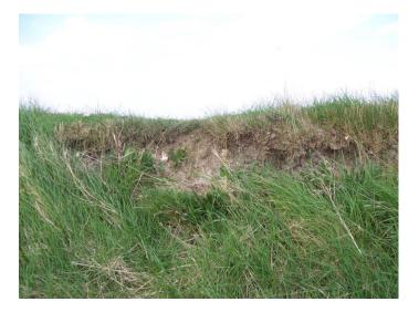
3. <u>Major repairs</u>. New development resulting from extensive repairs between Brick Dock and Aldeburgh Sluice to deal with slumped areas from Brick Dock to Aldeburgh Sluice. The works have resulted in some places with very steep back walls, loose earth through which grass has yet to establish and grow.
