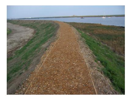
Photo at 456556 shows steep walls around the off river curve of e wall. It was in parts bald and steep before, now after repairs a better shape providing it can hold in heavy rain and with walkers. The bit just by here where the footpath also goes off at right angles across the marshes is still very steep if not steeper so may poach when wet.
