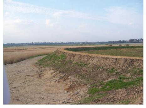
New pathway patchy, presumably where walls have been increased in height path has been restored to a width of 1.3metres but where the walls height was acceptable the path remains. See photo below ref 449563
