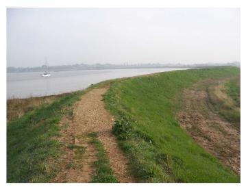
A 6. New concern that the landward face of the wall from West Row Point 445560 south east to 450554 is now showing a concave structure for some 100 yards. Does this mean it is slipping?
