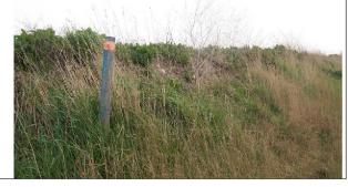
A.5 near vertical back/land ward slope of almost 1/5th of a mile of river wall TM445561 -449564. This is repeating the report last year as there has been no structural change in the wall but the waterlogged landward side base is of new concern as it is not a one off appearance as there has been no rain.
