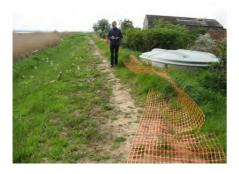
After Butley Mill Sluice No 2 at TM  $3858\ 5172$  the wall still has a clay surface. Tall grasses are beginning to grow through the surface.
