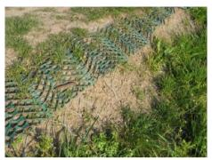
5. Small revetment collapse and an exposed steel reinforcing bar at the stile (TM 4241 4873). This was reported in 2012.
