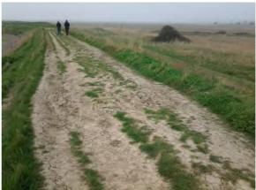
2. There is a significant dip either side of the manhole cover (TM 4233 4912) and where a path has formed down the inland bank
