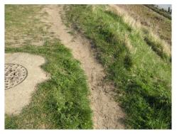
5. This year we stretched a taut string across in order to measure this dip. This shows that dip is 30cm lower than the adjacent river wall. The path to seaward is 45 cm lower.
