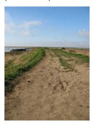
4. There is a significant dip either side of the manhole cover (TM 4233 4912) and where a path has formed down the inland bank. This has been reported in previous years. The right-hand photo shows erosion where a path has formed to seaward of the manhole cover.
