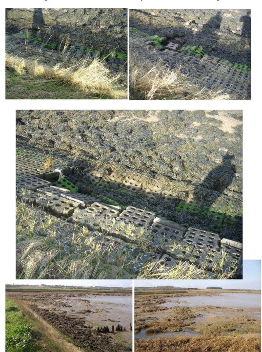
434 563 evidence of a mini slip just below the crest on the land side of the wall
