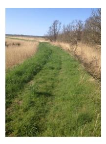
This area (photo above) which is at the north eastern end on Ham Creek wall was overtopped at the 2007 surge so must represent a slight lowering of the wall but there was no indication of subsequent damage to the wall.
