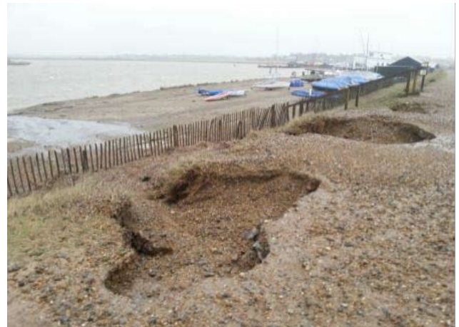
Large scour holes at the back of the shingle bank, 5 Feb 2014; source: Aldeburgh Yacht Club
