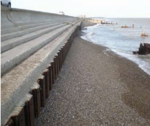
Exposed sheet piled toe at Slaughden, south of Aldeburgh town, 26 February 2014; source: Environment Agency
