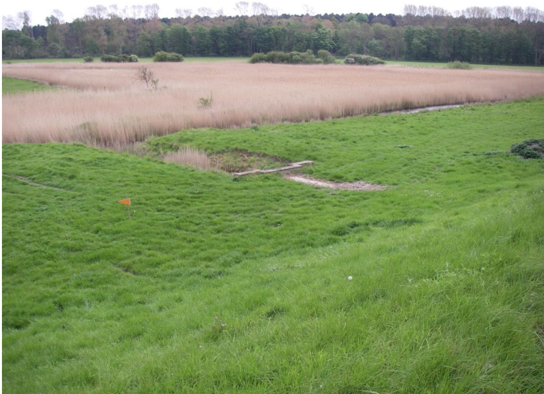
View south east from Ch 750m. Head wall of old sluice will restrict access during earthworks.
