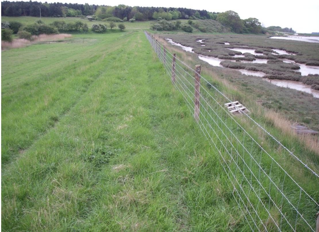
Looking south from Ch. 200m showing levee merging into higher ground. Note quality of grass, this is sheep grazed.
