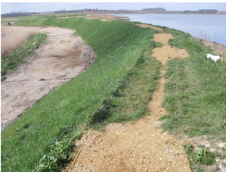
View looking south west from Ch 2900.
