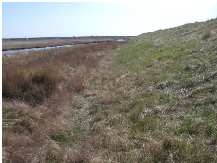
View looking east from Ch 500.
