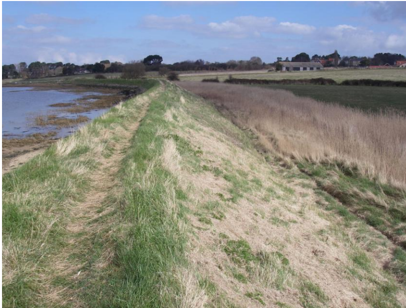
View looking north north west from Ch 3200.
