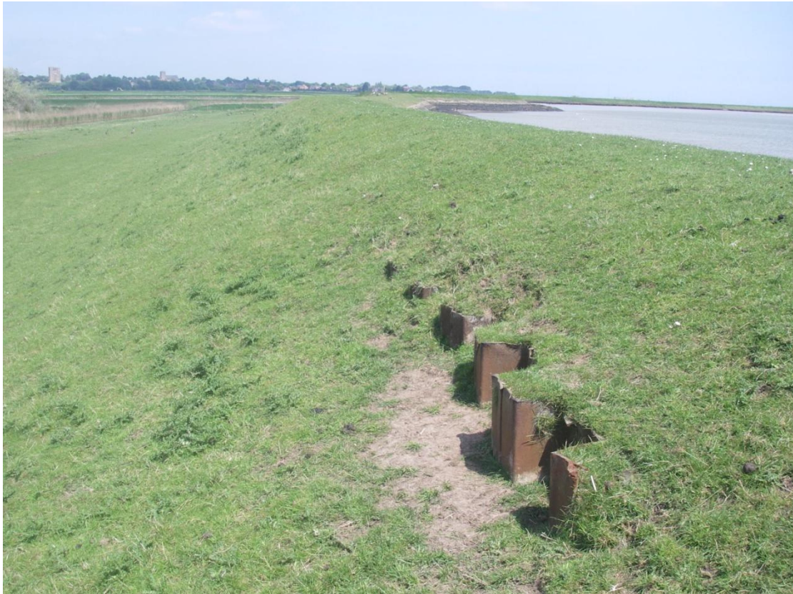
View north east from Ch 4200 showing dead men anchoring for pile wall along the seaward side of the levee.
