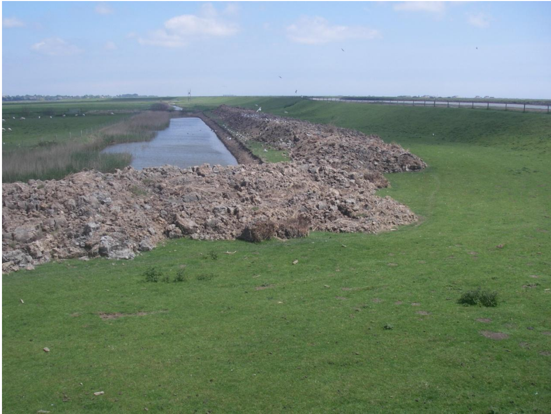
View north east from Ch 2800 showing borrow ditch and windrowed clay drying for use in levee.
